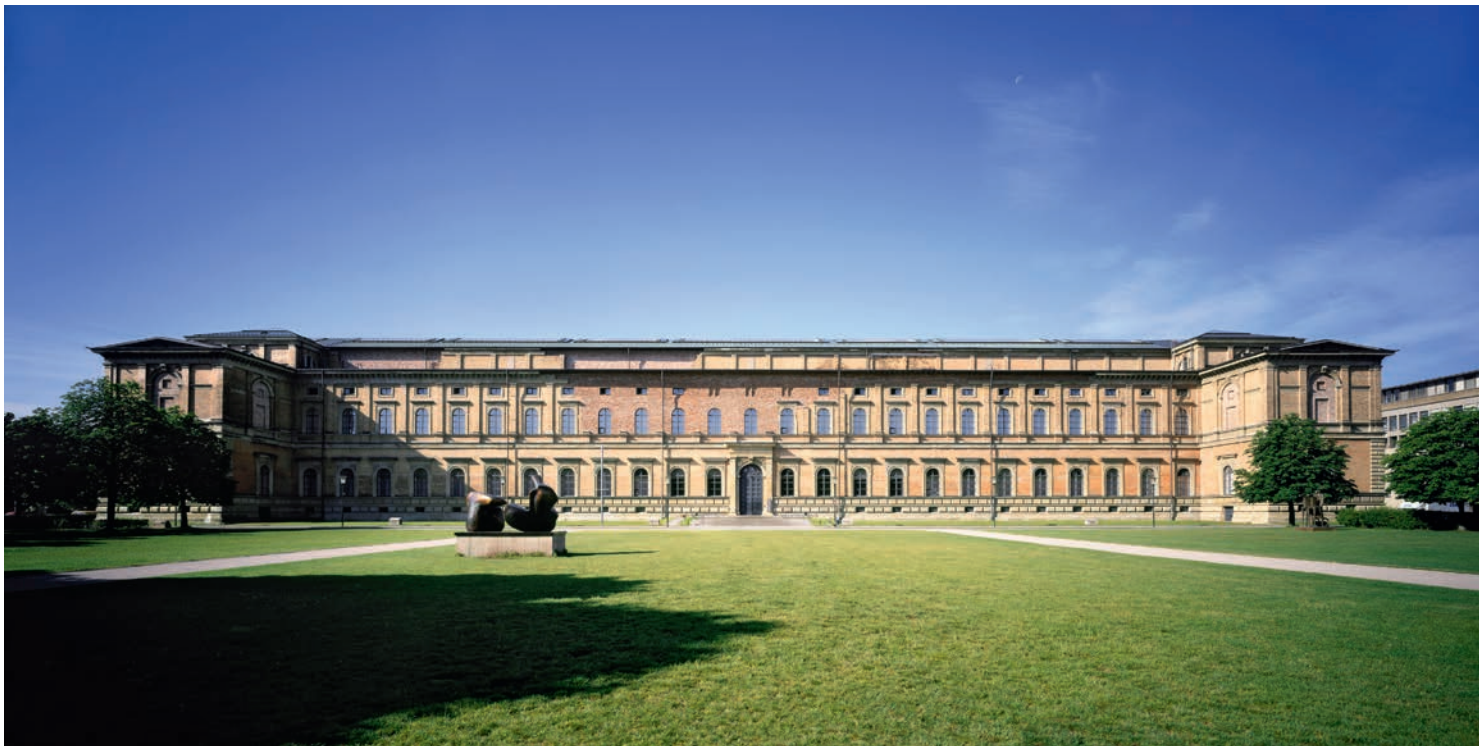
FIGURE 1 Munich, Alte Pinakothek, north façade with today's entrance
